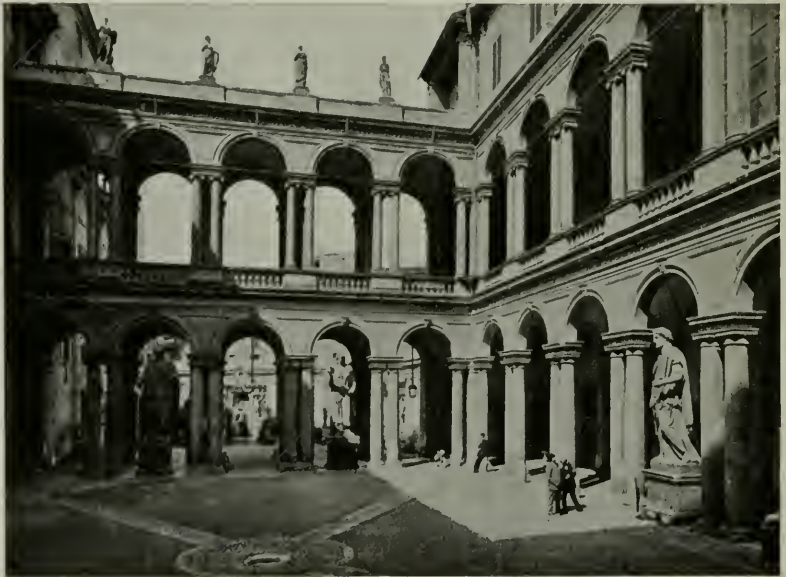
CORTILE OF THE PALAZZO BORGHESE, ROME.
